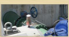
G-LUBE EM B ensures precise lubrication for up to one year and is is completely self-sufficient due to its operation on batteries. Thanks to the high operating pressure, it can also be used for several lubrication points if required.
